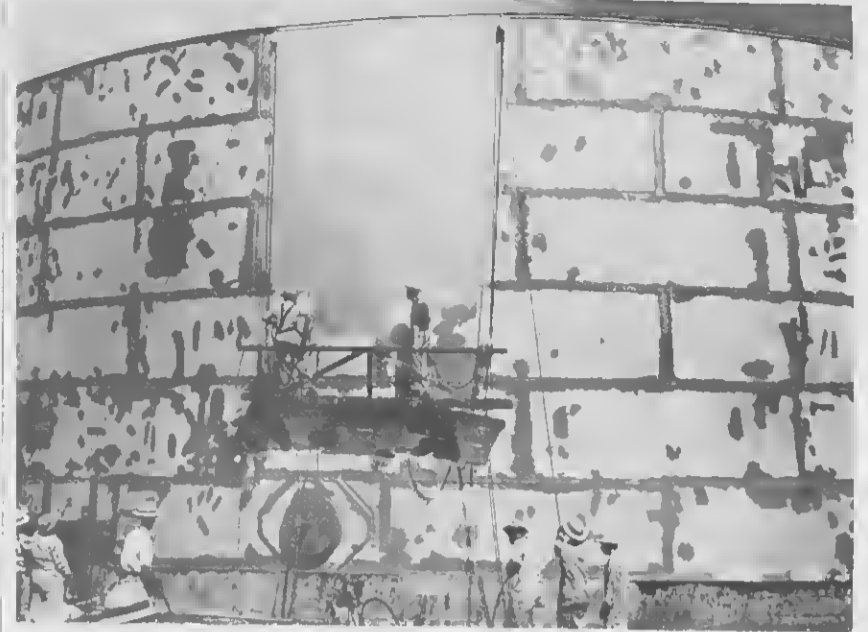
PAINT CREWS test the new DeVilbiss paint spray on a tank. Teams of three painters each tried out the spray.
